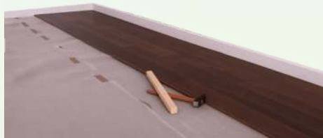
WOODEN FLOORING UNDERLAY
